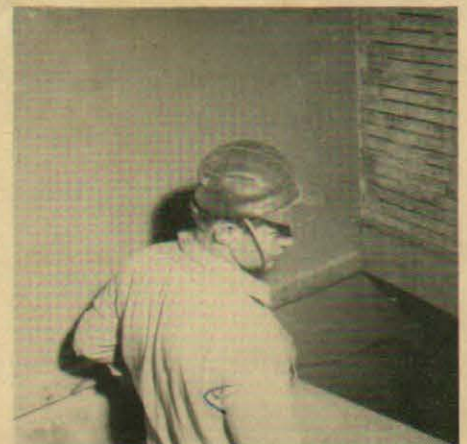
Carpenter at work at Marstellar residence.
